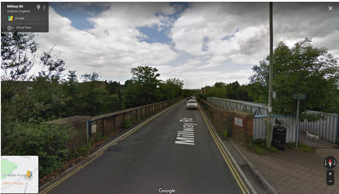
View looking North over Millway Bridge.
